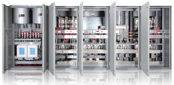
Rear view of SuperSwitch 4000A showing system modularity
